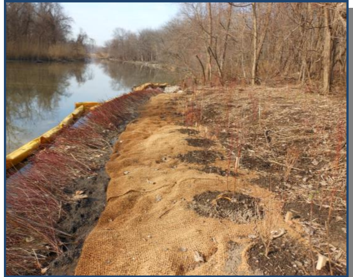
River bank restoration utilizing bio-engineering techniques
