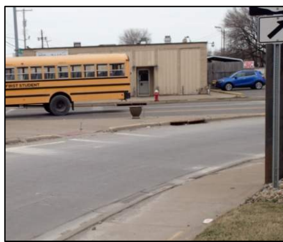
Photo 6: Faded Crosswalk Markings at Kansas Avenue /Colorado Avenue Intersection
