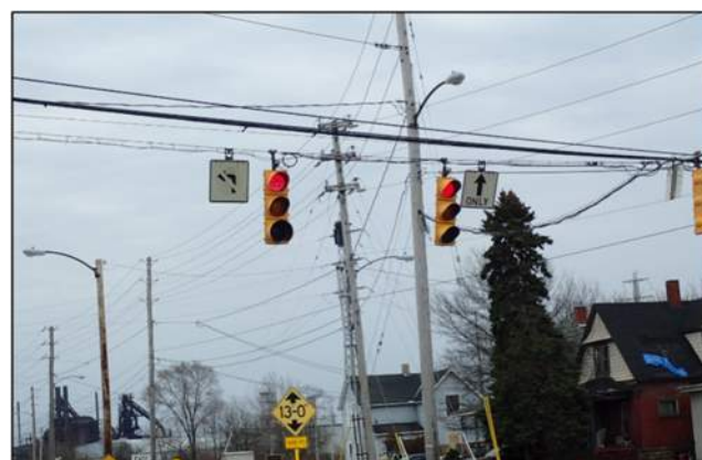
Photo 11: Faded Turn Lane Signage at SR 611 and Elyria Avenue
