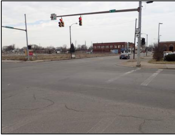
Photo 16: Faded Crosswalk Markings at SR 611 and Broadway
