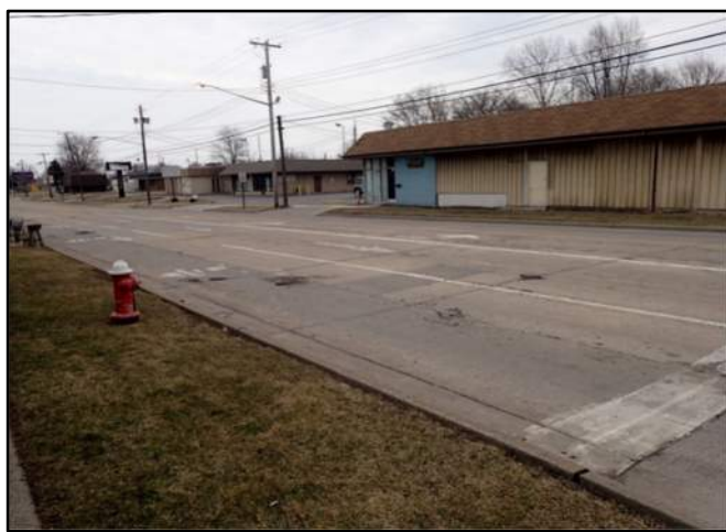
Photo 5: Faded Pavement Markings at Kansas Avenue /Colorado Avenue Intersection
