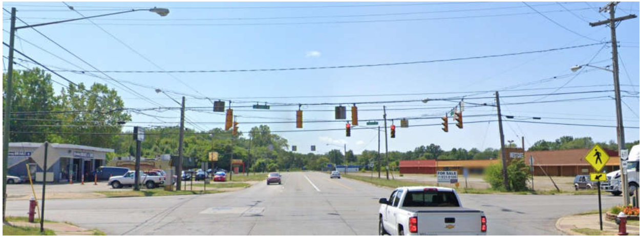
Figure 4 - Westbound Intersection Approach - Courtesy Google Street View
