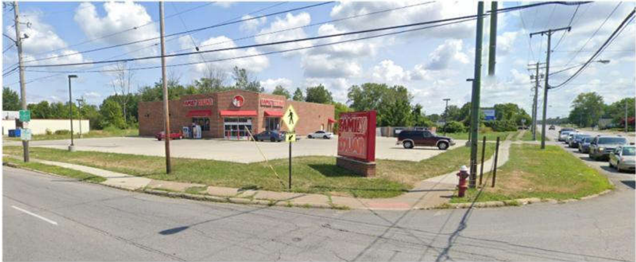
Figure 2 SE corner of intersection - Courtesy Google Street View
