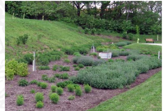
Bioretention Cell Image: Ohio EPA Rainwater and Land Development Manual
