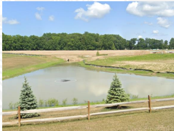
Wet Extended Basin at Cornerstone Farms During Construction Image: © 2023 Google
